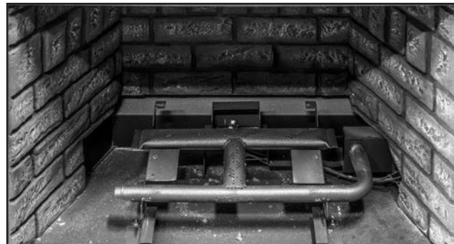
Figure 50: Remove the 6 screws highlighted in figure 49 using a Torx T-20 screwdriver and remove the air deflector
